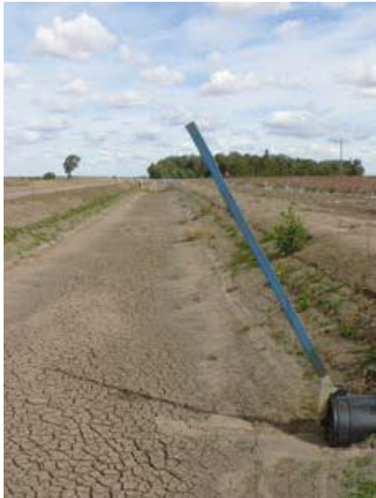
Fig. 3: Manually operated PTB (Source: Wood and Carrigan 2006)
