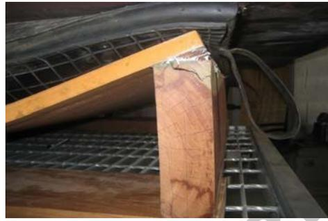
(b) Joist cracking
