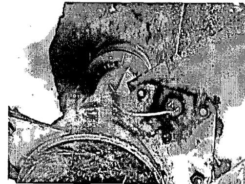
Fig 2. Acoustic transducer located in a flange of the primary extractor fan
