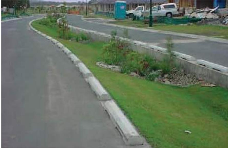
**Figure 1.5** Photograph of a bioretention swale in Melbourne
