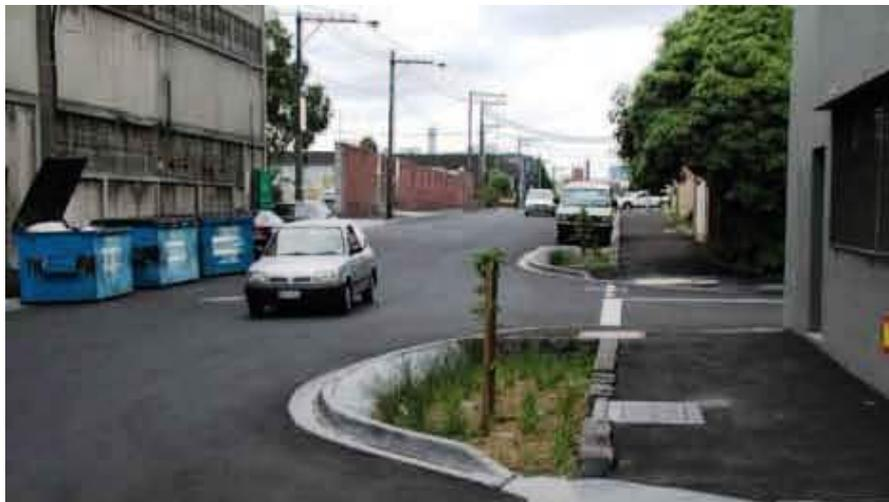
**Figure 1.3** Photograph of a bioretention basin in Melbourne
