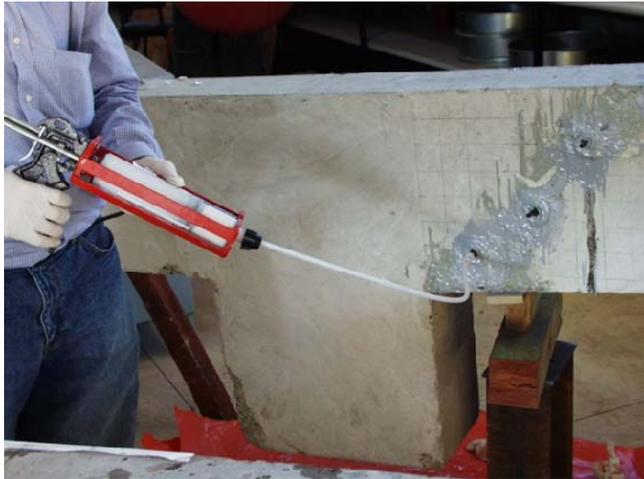
**Fig. 4. Repair of the Shear Crack by Epoxy Injection**
