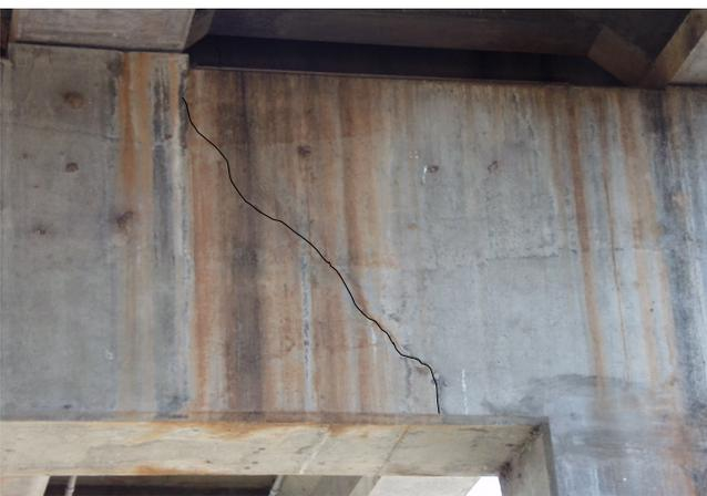
**Fig. 8b. Crack in Tenthill Creek Bridge Bent Cap (location highlighted)**
