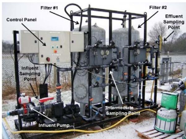
Fig 5: Unit processes of Filter Pairing A.
