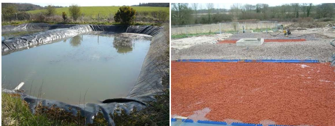
**Fig 1:** Tertiary settling pond at Wessex Water's Cranborne WTP prior to retrofitting (left); the same settling pond after installation of the technology (right).
