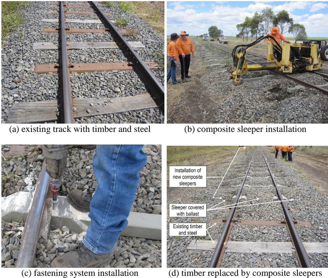
Fig. 5: Installation of composite sleepers replacing existing timber
