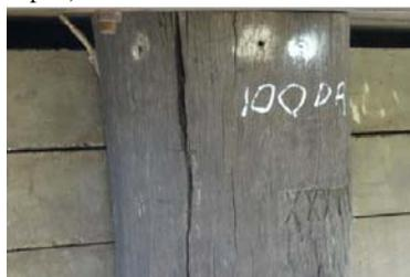
(e) Vertical splitting (overloading-top of pile)
