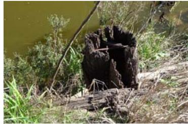
(c) Severe rot and pipe (wingwall pile)
