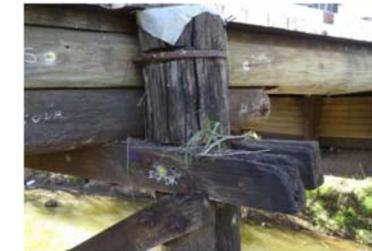
(f) Vertical splitting (changed section-top of pile)
