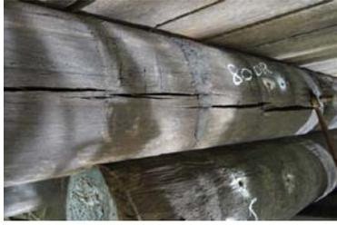
(a) Splitting (girder with a fastener)
