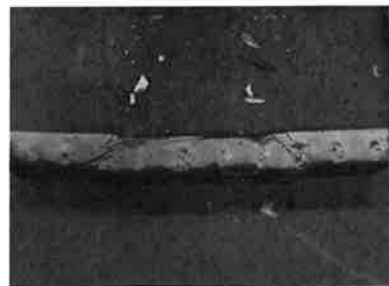
Figure 4b. Cracking pattern of specimens with BS50
