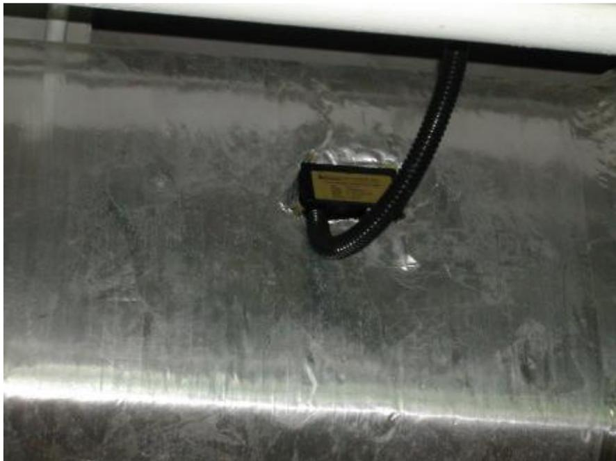
Figure 5.5 Duct Static Pressure Sensor
