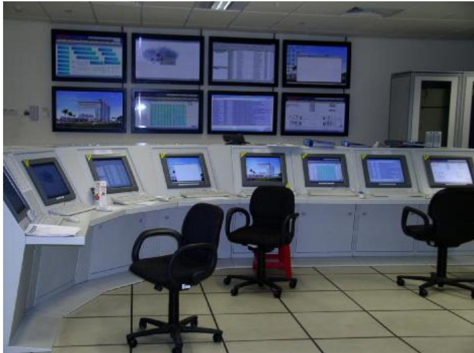
**Figure 4.1 Intelligent Building Management System (IBMS) Control Room**
