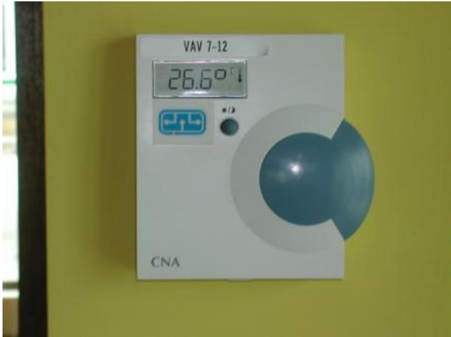
Figure 5.4 VAV Thermostat
