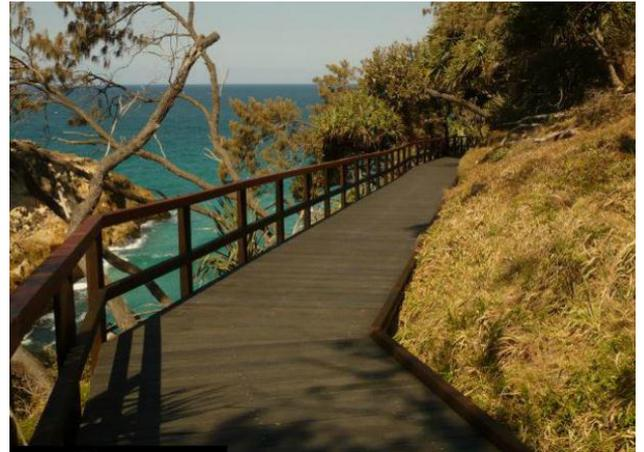
Figure 6. Composite sandwich boardwalks.
