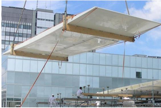
Figure 11. Lightweight GFRP sandwich roof [24]
