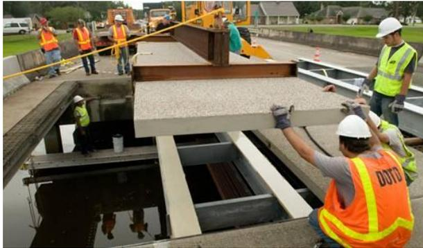
Figure 4. Balsa-cored composite bridge deck [13].
