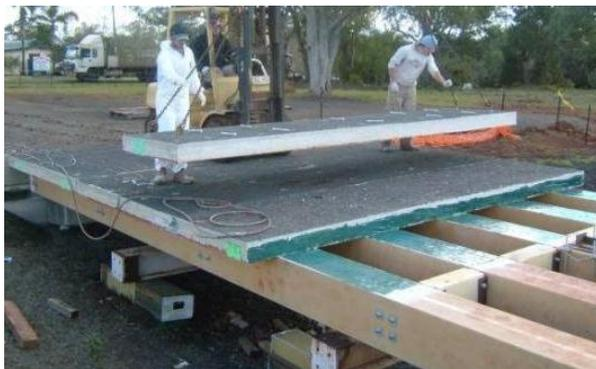
Figure 8. FRP sandwich bridge beams at USQ.
