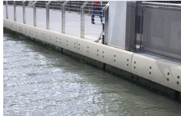
**Figure 5: Fibre composite reinforced waler**
