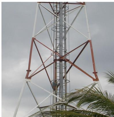
Figure 1. Steel trusses in communication tower
