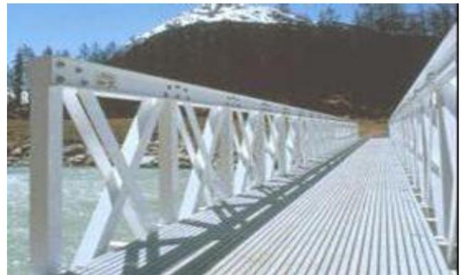
Figure 4. The all FRP composite Pontresina bridge (Keller et al. 2007)
