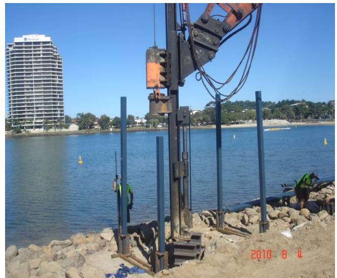
FIGURE 01: Application of composite pile.
