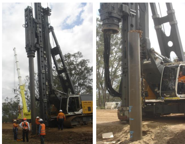
FIGURE 02: Pile driving rig for trial test.
