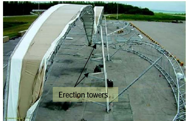
Figure 2: B2 Shelter during erection
