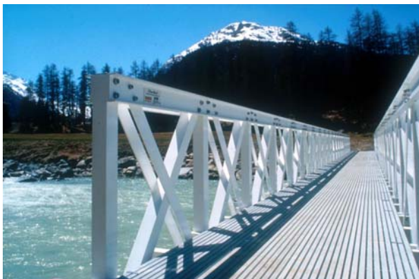
Figure 3: Pontresina Bridge, Switzerland
